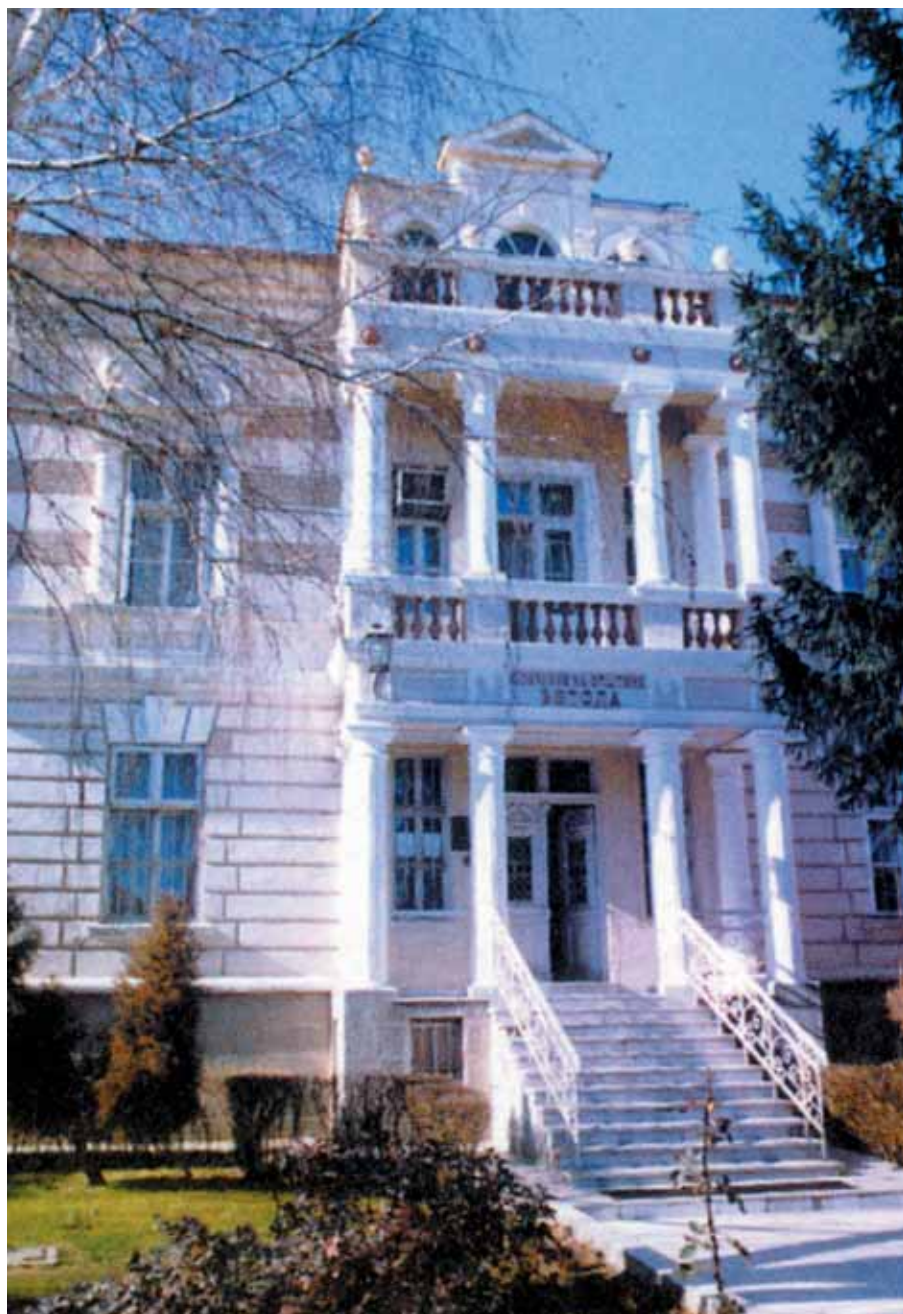
Figure 72. The former Greek Consulate-General in Monastir
