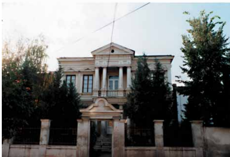
Figures 86, 87. Mansions: Above: The house of the Xyftas family Below: The Makalis house
